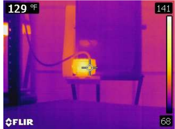
The motor having the exterior temperature show over 130F means the inside is even warmer. This could be a sign the motor is toward end of life, or be slipping.
